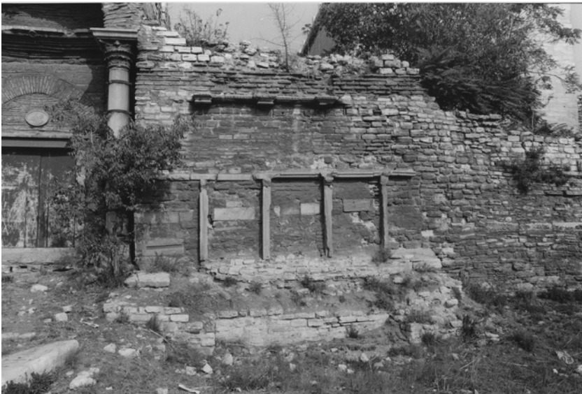
Fig. 12.2. The Golden Gate of Constantinople's triumphal outer gate: south curtain wall, showing tiers of frames.
